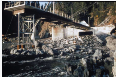
Dock on Hinchinbrook Island, Prince William Sound, Alaska uplifted 8 feet during the 1964 M9.2 Alaska earthquake. USGS photograph.
